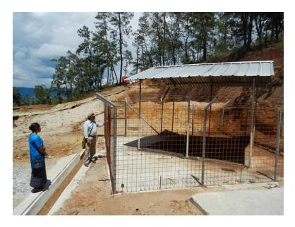
Down the mountain ridge from the entry to the Los Coches tunnel, we pass one of the "respiradoras" – a sort of huge chimney / exhaust tunnel, over 6 feet in diameter, that releases exhaust of contaminated airs from the tunnel far underground.
