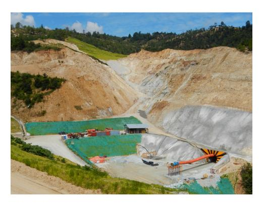
A few years ago, Goldcorp clear-cut the forest at this 'Los Coches' pit and then used explosives to blow up and remove the mountain, layer by layer. This mountain-top removal technique is used, generally, when the gold is minutely dispersed in the earth and rock. The entire mountain of rocks and earth, blown up and crushed, is then processed in Goldcorp's plant, half a mile down the mountain, using cyanide and other chemicals to separate the gold from all other minerals.
