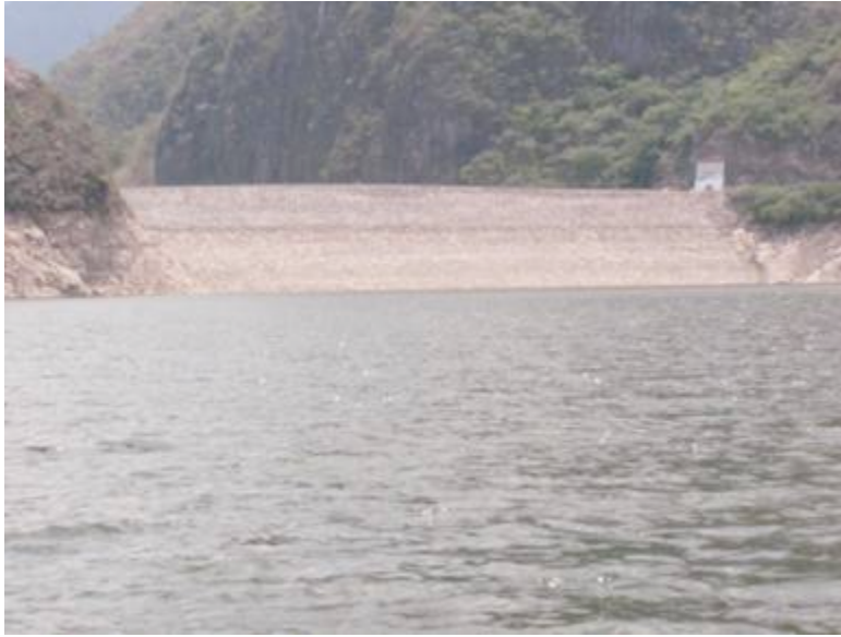
(The Chixoy dam wall, seen from up-river, on the flood basin. The remains of a number of the illegally evicted communities lie deep below the water. Photo: Rights Action)
